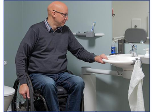
Sinks should be fitted at a wheelchair users height of 720mm-740mm, to allow a person to be able to position themselves as close as possible.
