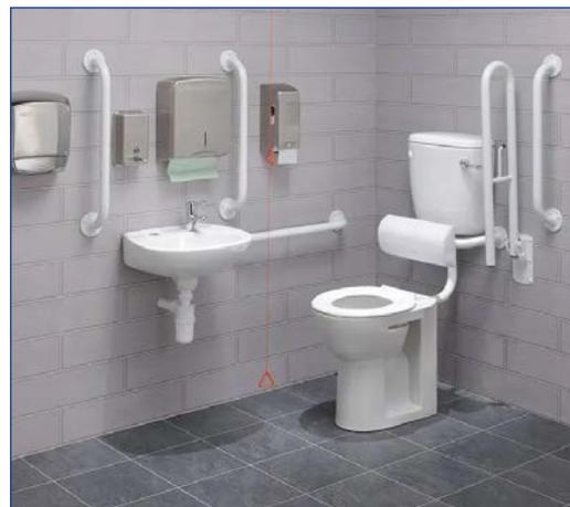
It is recommended that accessible toilets should measure at a minimum 2.2m length by 1.5m wide. The height of an accessible toilet must be between 440mm to 500mm. Accessible toilet fixtures and fittings (such as changing tables and frames) should be always be kept clear of the manoeuvre and transfer spaces to prevent obstructions.
