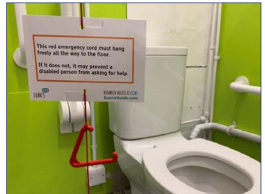
Emergency cords must be positioned between the toilet and transfer space. The handle of the emergency cord must feature a triangular design, so that it is easier to grip and grab.
