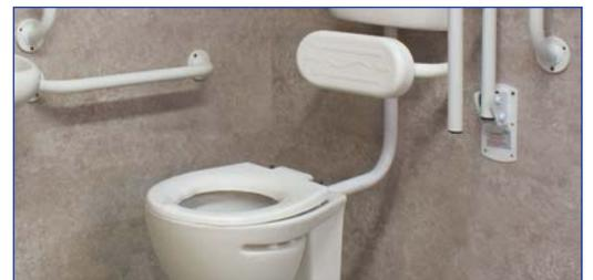
Both right and left hand transfer should be available where possible, where not possible the use of an angled lateral transfer toilet should be applied. Obstructions to legs and footplates must always be avoided.
