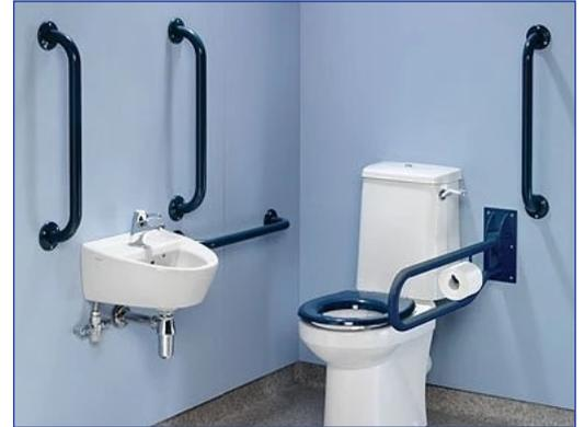
There should be a minimum of 5 grab-rails available. Grab rails must be properly secured with stable substrates and fittings to prevent accidents when weight or pressure is applied with a persons body weight.
